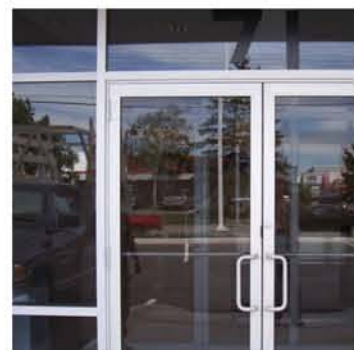
7 storefront system - clear anodized aluminum
